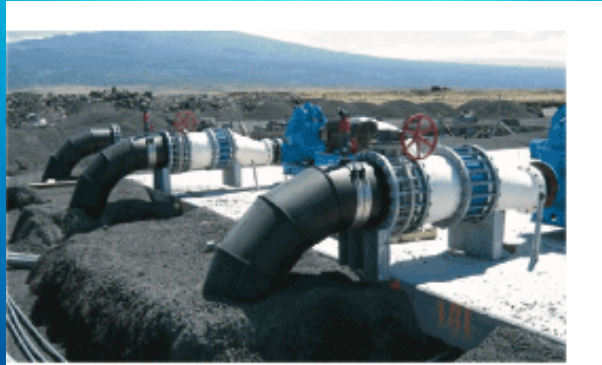
The pumping station
